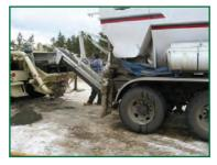
Another challenge for this project was the concrete delivery and placement. The closest batch plant is 18 miles away, and the slow climb to the site makes the travel time over an hour and fifteen minutes long. Advantage Exteriors decided to utilize a site-mix concrete company called 24/7 Site Mixed Concrete, who would load
