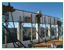
The construction of the main floor was relatively simple compared to the extraordinarily difficult foundation phase. The walls, which are twelve feet tall, have numerous large windows to utilize the abundance of natural light and capture the stunning views. They also provide support for the second story.
