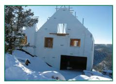
the top nineteen feet. As that top gable was poured, stops had to be created within the wall so that the pump could continue to place concrete all the way up to the peak.
